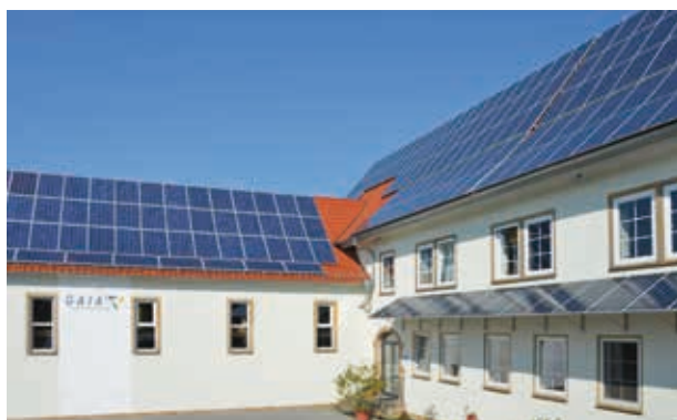
GAIA company headquarters: an energy-generating old building with exemplary character
